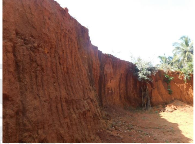
Photo 13: Soil profile section of Vertical Slope Cut in the study area.
