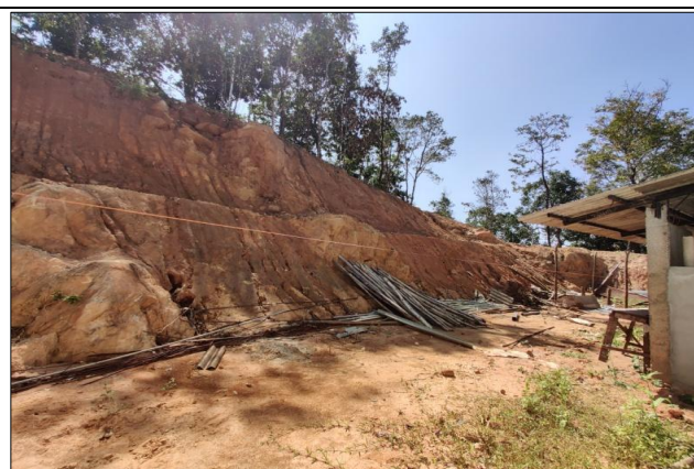
Photo 7: Extensive Cut Slope failure on lowly dissected hillslope in Ganapatikatte Village of T.S. no. 480/6
