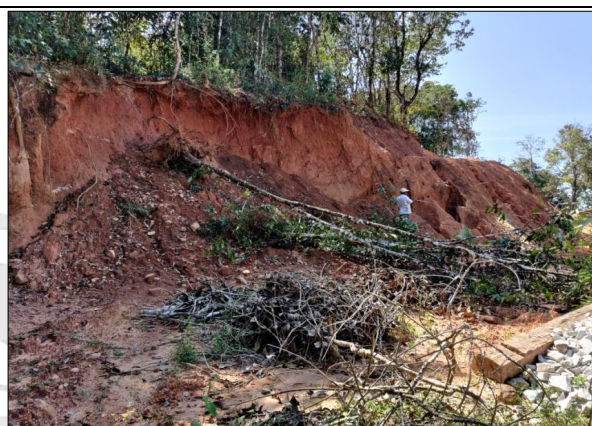
Photo 7: Extensive Cut Slope failure on lowly dissected hillslope in Ganapatikatte Village of T.S. no. 480/6
