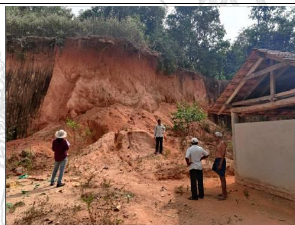
Photo 9: Settlement on Modified Slope Nagalapur Village of T.S. no. 480/6
