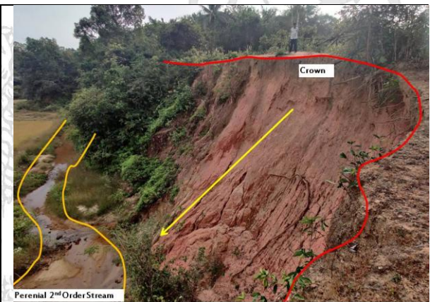
Photo 4: Debris Slide South of Kalgudge Village/Koppa road at 13^{\circ}35'48.4''\text{N} / 13^{\circ}35'48.4''\text{N}
